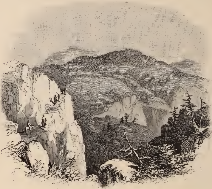
ROAD CUT IN THE ROCKS.
